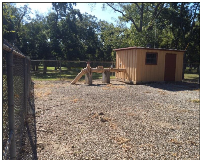
Figure 1: Existing Well 19 Pumphouse and Piping
